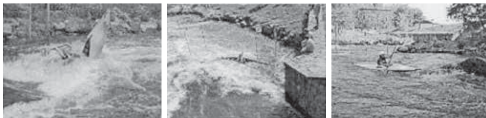
Abb.: White Water Slalom Ceske Budejovice, Artificial Slalom Waterway Length of the waterway: 610 m, Altitude difference: 5 m, Flow of water: 0-25 m 3 /sec.
